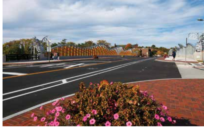
Figure 4. Approach to the bridge showing widened sidewalks.
