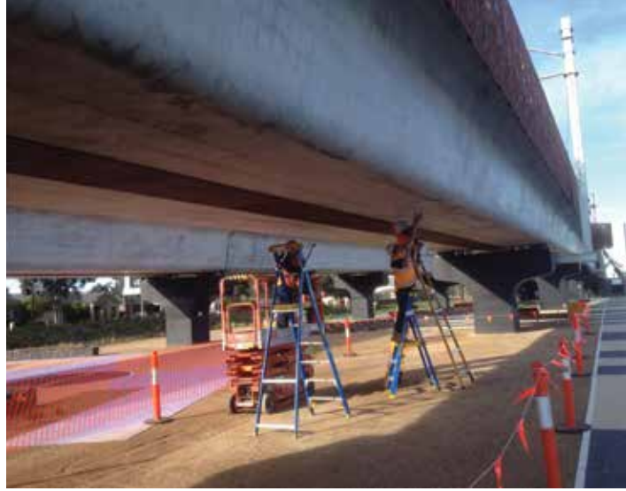
Installation of the PARC MOXI smart monitoring system on one of the VicRoads' bridges in Victoria, Australia. Based on fiber-optic (FO) sensors, MOXI accurately estimates parameters indicative of the bridge health state.
