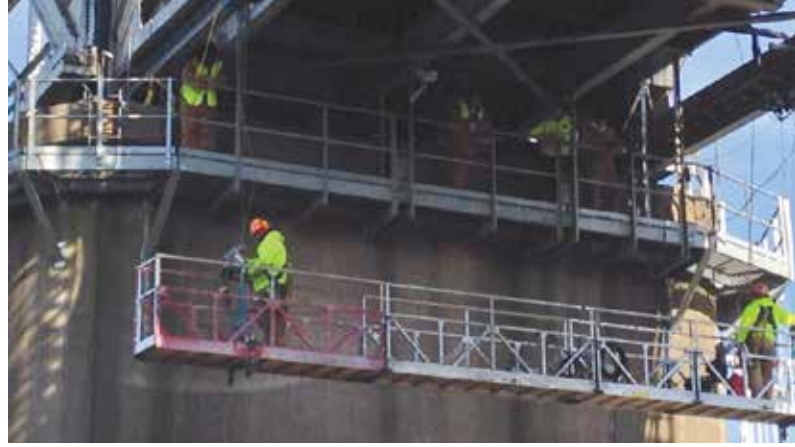
Traveler rail retrofitted to accommodate a scaffold system for inspections.
