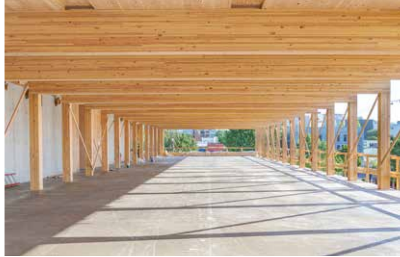
Long-span glued laminated timber beams.
