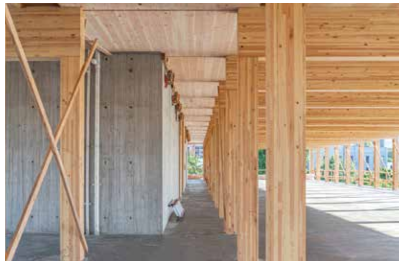
Central colonnade at concrete core.
