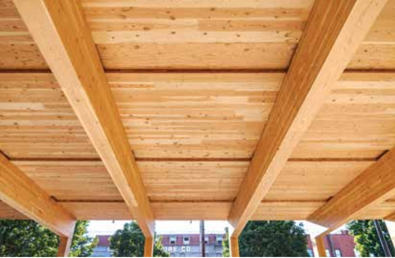
CLT chases over glulam beams.
