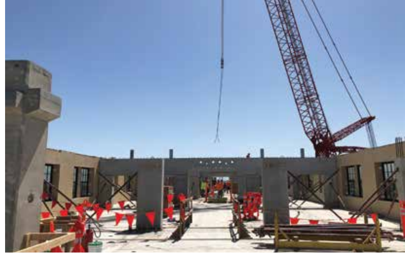
Transverse moment frame erection.
