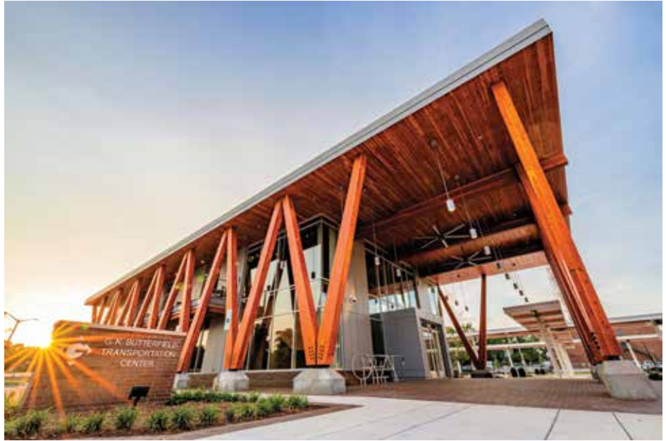
Cross-laminated timber was utilized as the roof diaphragm and shear walls at the G.K. Butterfield Transportation Center in Greenville, North Carolina.
