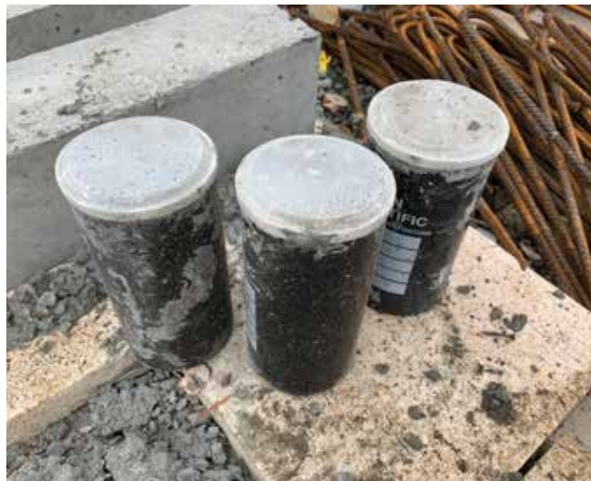
Field-cured cylinders, onsite.
