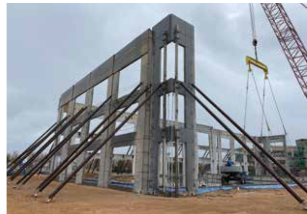
3-story tilt-up panel braced to the exterior using temporary helical piers.
