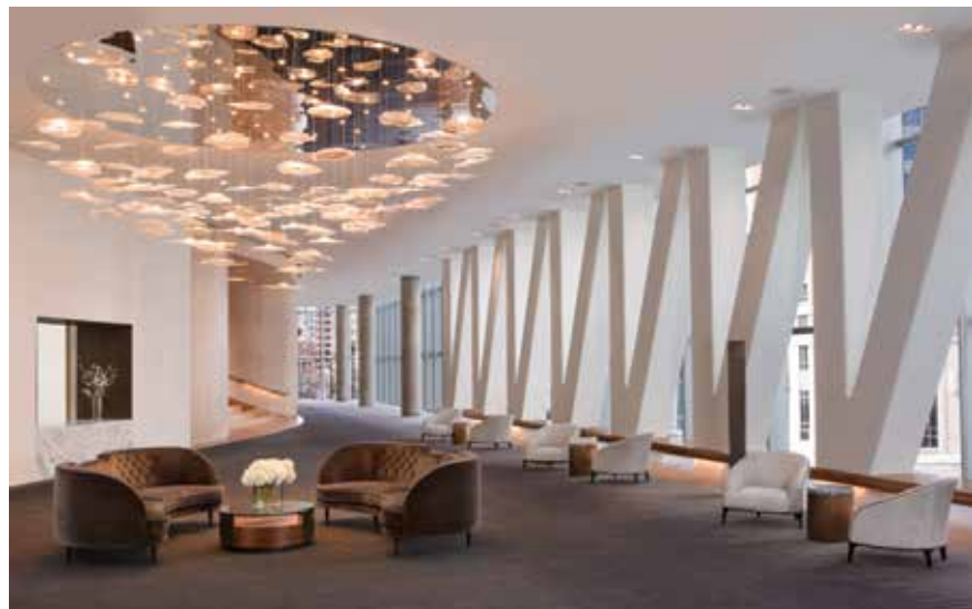
Figure 5. Truss spanning over porte-cochere and supporting the green roof above within the completed prefunction space. Courtesy of Sammy Todd Dyess.
