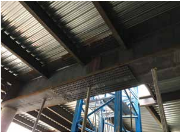
Figure 3. Transfer girder splice.
