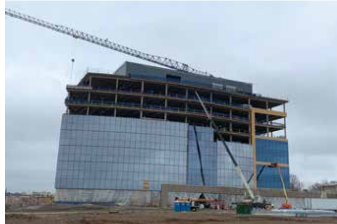
Shamrock Trading Project w/A913 beams, Overland Park, Kansas.
