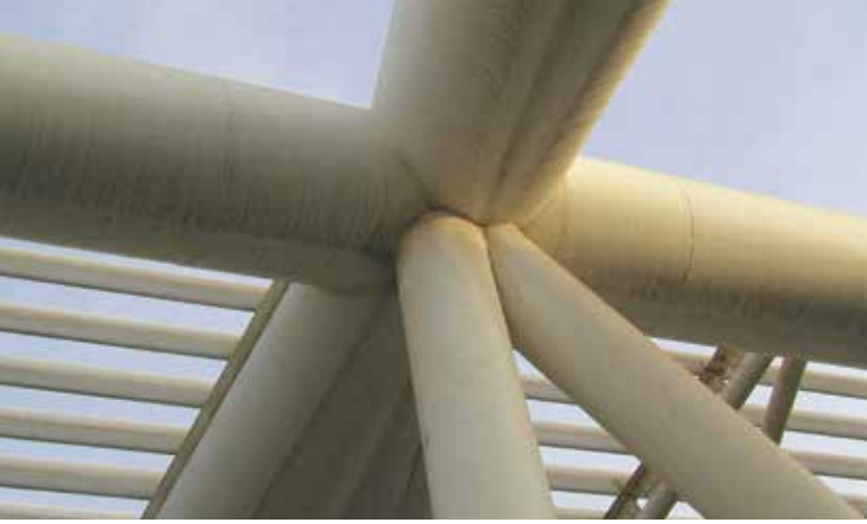
Figure 2. Complex end profiling.
