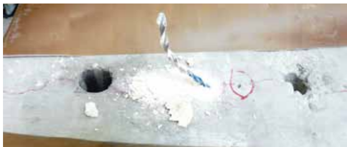
Anchors tested to shear failure showed localized crushing in the limestone in shear. Courtesy of Specialized Testing Inc.
