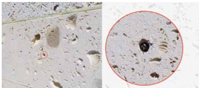
Countersunk anchors blend in with natural voids on the stone surface.
