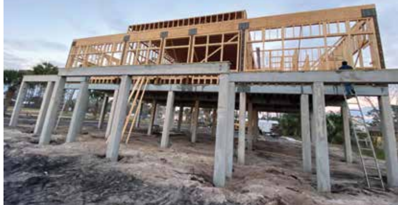
Performance-based design utilizing a moment frame to maximize openings on a new coastal home in Port St. Joe (Gulf County).
