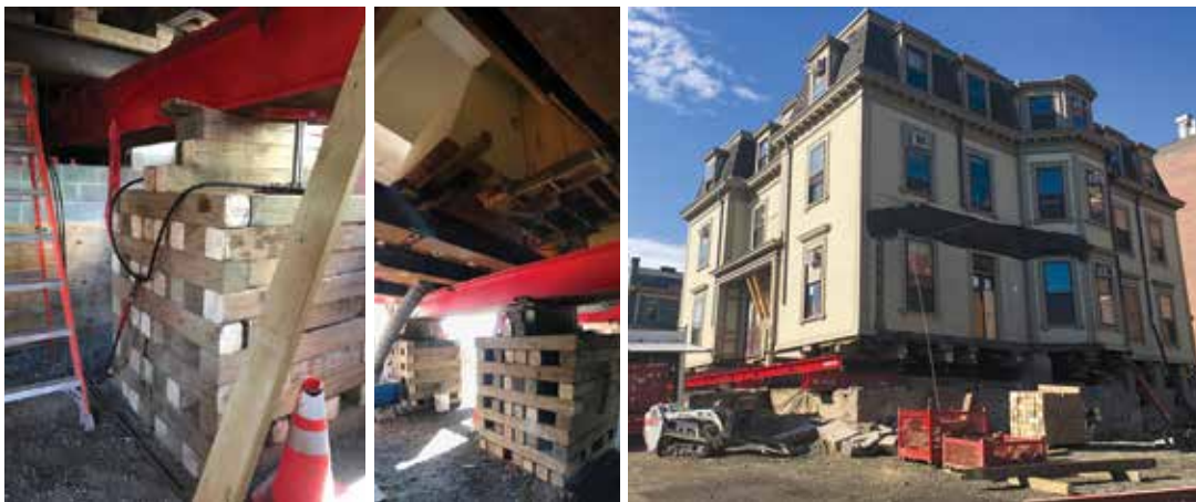
Figure 4. Hydraulic jacks (two left photos); Gridwork of cribs (right).
