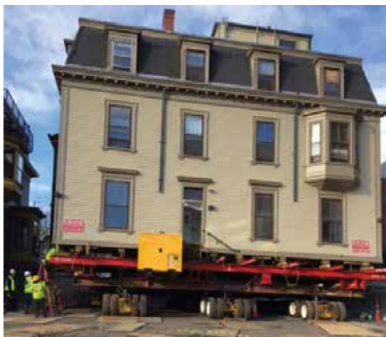
Figure 5. On the move, with dollies in place.
