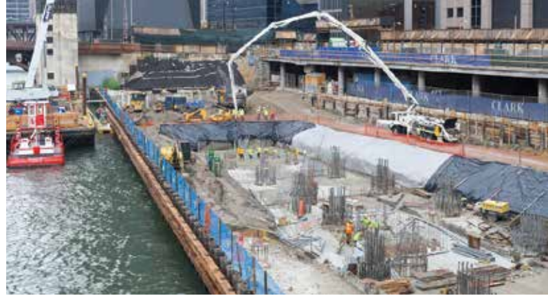
Site looking north. Mud-slab placement in advance of mat slab pour (3,300 cubic yards placed in less than 8 hours) for the building core. Reinforcement projections include interior "bar cassettes" and exterior circular bars.
