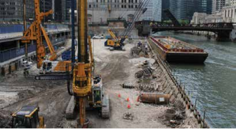
Site looking south. Upper and Lower Wacker Drive to the east (left). The barge moored to the Chicago River Wall provided laydown areas for material storage and a platform to tie reinforcing cages.
