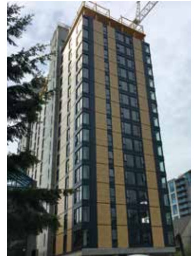
Figure 1. Brock Commons-Student Housing, Vancouver, BC. Currently the tallest mass timber building in North America at 18 stories.
