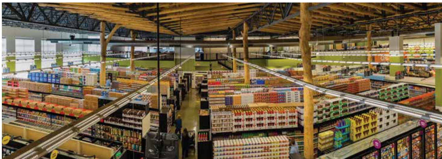
Figure 5. Festival Foods Grocery Store (Madison, WI). The red pine SRT trusses span up to 55 feet and support up to 500lbs/lf. The load-bearing Ash Columns support up to 220kip in live and dead loads. Courtesy of Heartland Photography.
