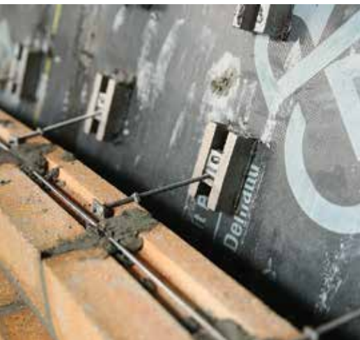
Figure 4. The custom brick tie system.
