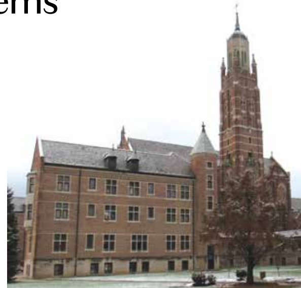
Figure 1. Masonry Bell Tower.
