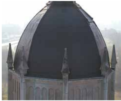
Figure 2. Drone image of the top of Bell Tower.
