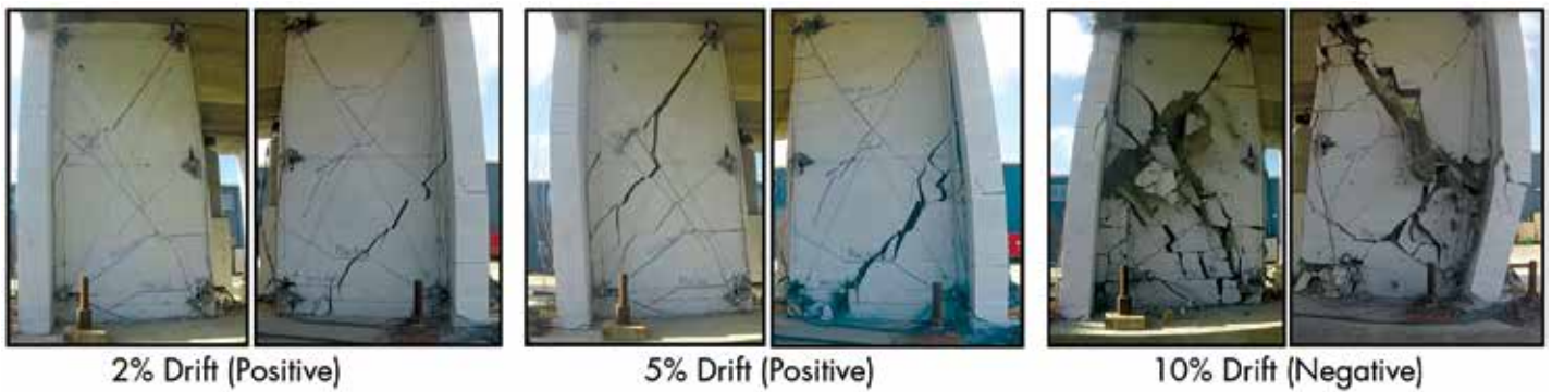
Figure 3. Damage in the T-walls of Specimen 2 at different roof drift levels.
