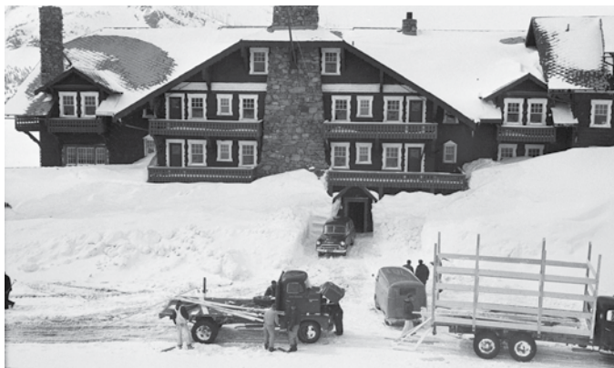
The Many Glacier Hotel in April 1956. Snow has reached the second floor of the lobby. Chimney at left was removed at an unknown date before the recent rehabilitation work. Courtesy of Glacier National Park Archives.
