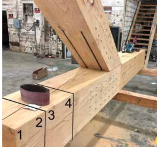
Figure 8. Mockup of the typical bottom chord connection, which led to fabrication adjustments.
