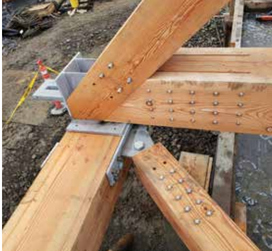
Figure 7. Final connection in progress at concrete abutment not yet placed.
