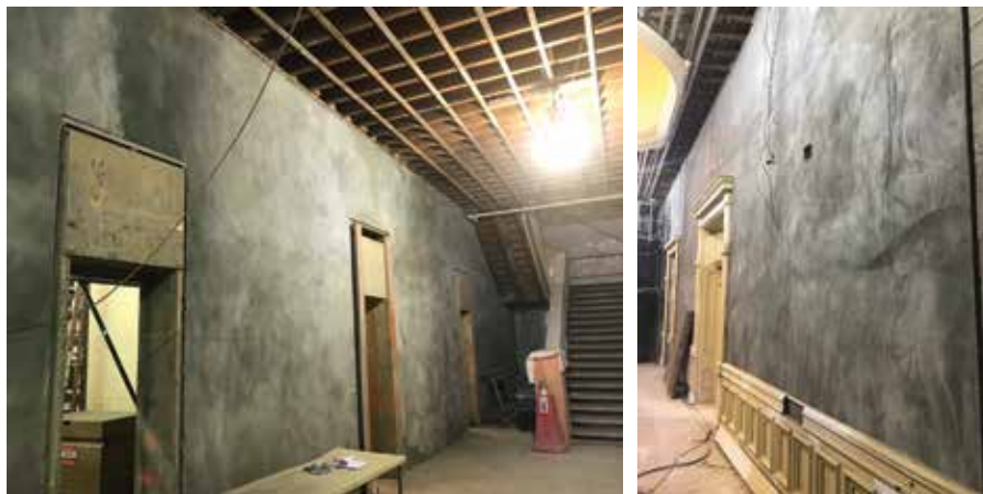
Figure 6. Finished FRCM installation on first floor (left), second floor (right).
