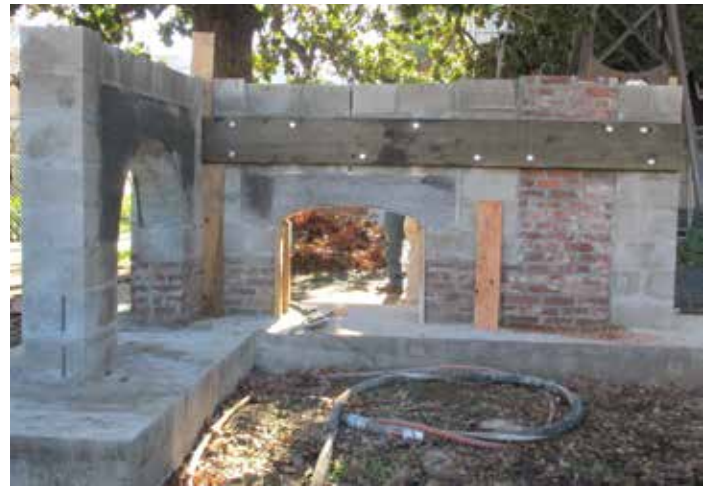
Figure 3. Mockup prior to installation of FRCM.
