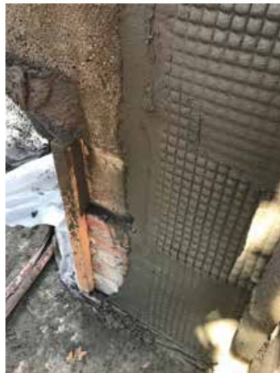
Figure 4. FRCM fabric being installed into matrix.
