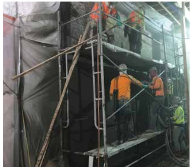
Figure 5. FRCM installation.
