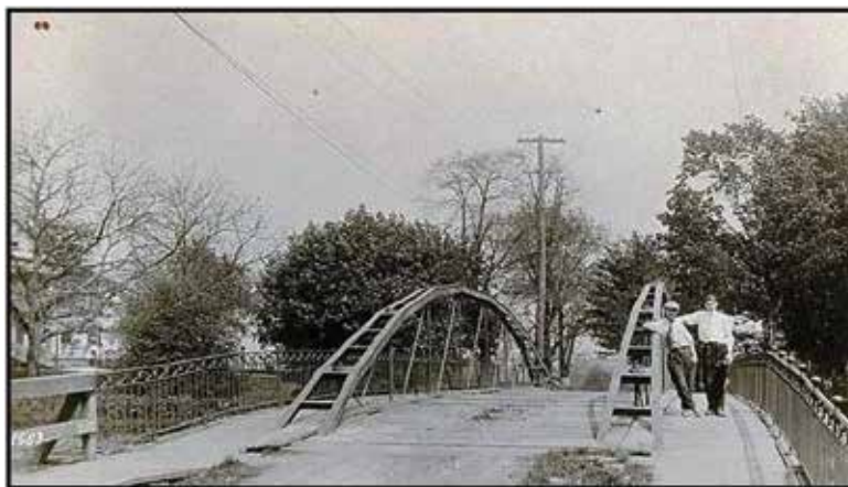
Whipple Bridge at Holley, NY, built at the same time as the Albion Bridge.
