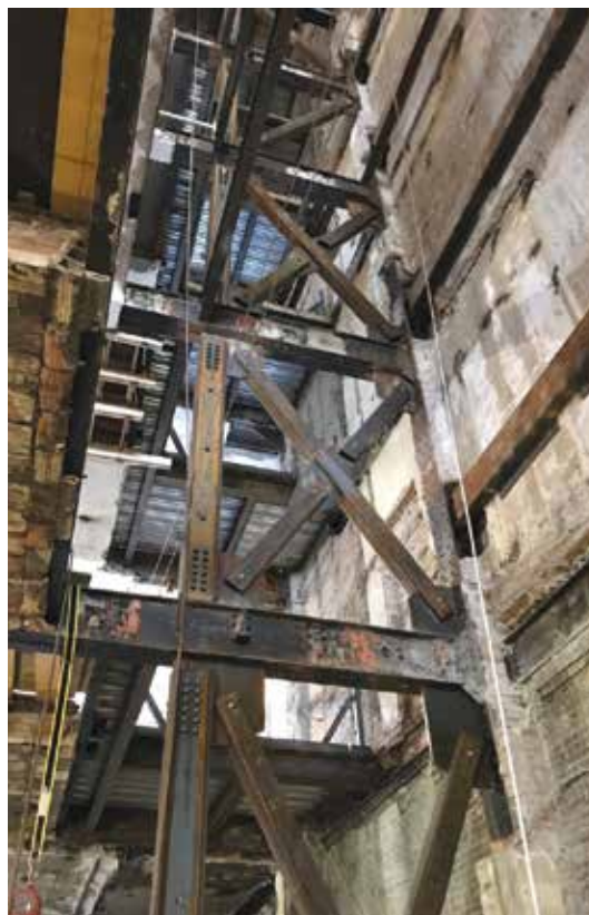
Figure 2. One of three new braced frames erected in the existing building.
