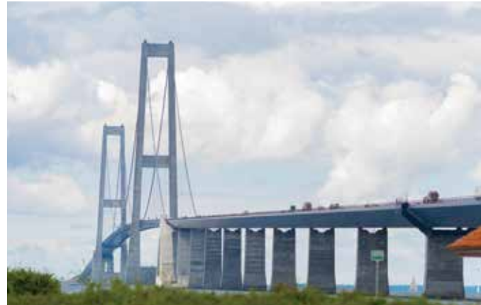
Great Belt East Bridge, Denmark.
