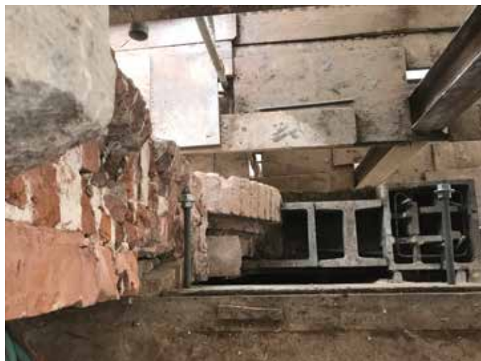
Figure 5. Detail of CMU interface with historic brick arch.
