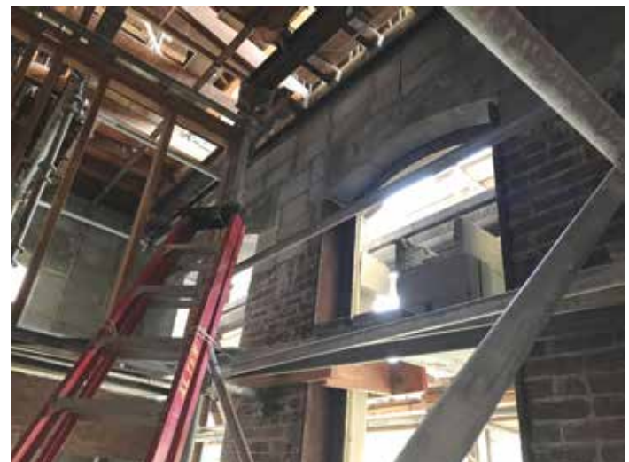
Figure 6. CMU and precast lintel construction above the original brick wall.
