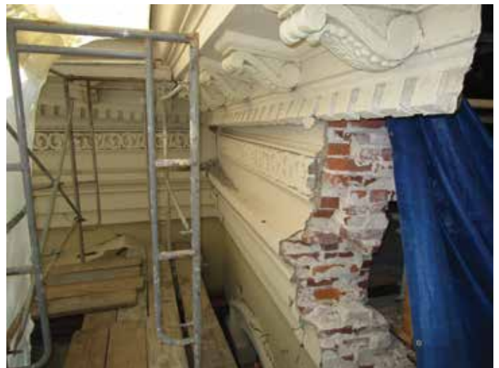
Figure 2. Historic exterior wall brick construction and dental cornice.
