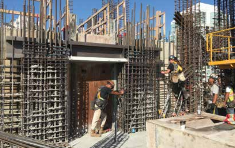
Wide-flange coupling beams in construction.
