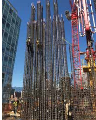
Vertical post-tensioned high-strength DYWIDAG threaded rods in construction.
