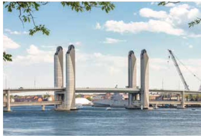
FIGG and Hardesty & Hanover were Award Winners for the Sarah Mildred Long Bridge project in the 2019 Annual Excellence in Structural Engineering Awards Program in the Category – New Bridge and Transportation Structures. Photos courtesy of FIGG.
