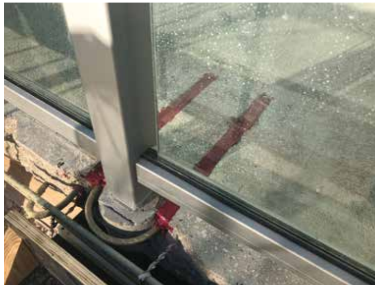
Figure 4. GFRP hairpin installed around a railing post grout pocket.
