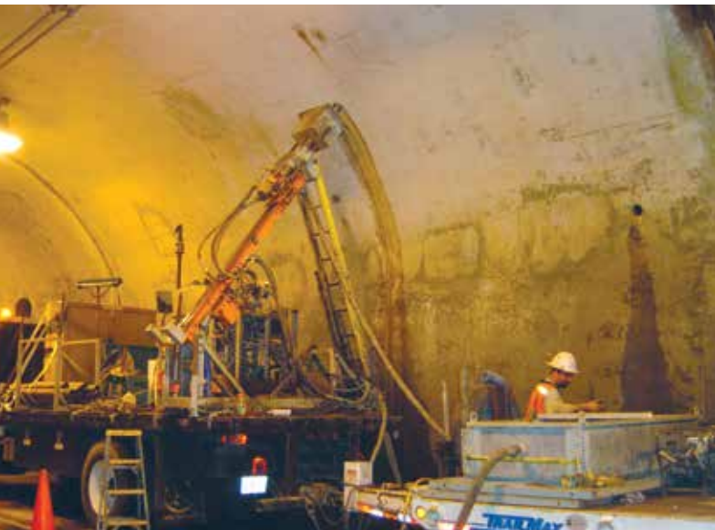
Specialized rock coring equipment for explorations within an existing tunnel.
