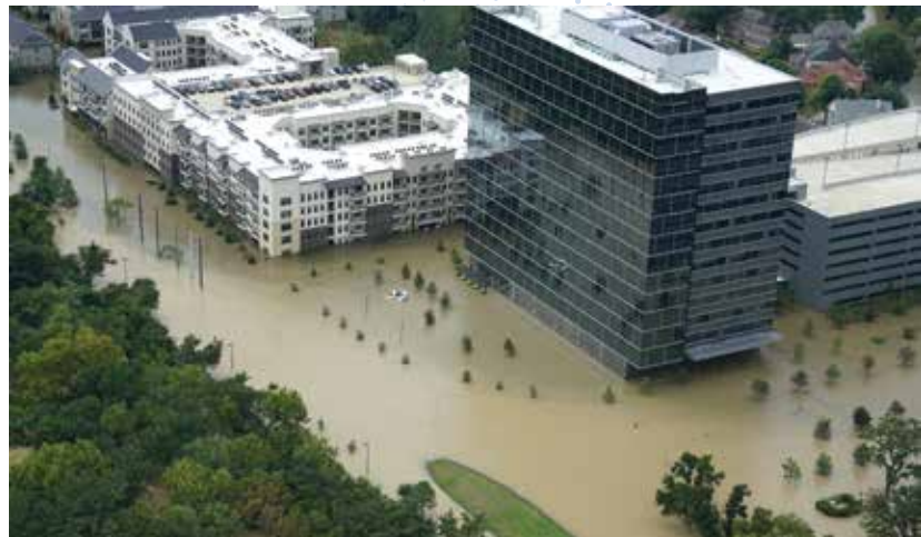
Figure 1. Flooding caused by Hurricane Harvey's massive, persistent rain resulted in $125 billion in damages and 65 deaths across the Houston region and Southeast Texas in 2017. Courtesy of ThinkStock.
