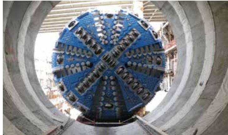
Figure 1. Pressurized tunnel boring machine.
