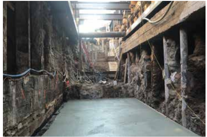
Figure 4. Urban excavation abutting existing tunnel (left) and other structures.
