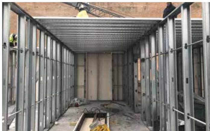
Unshored composite steel deck construction.
