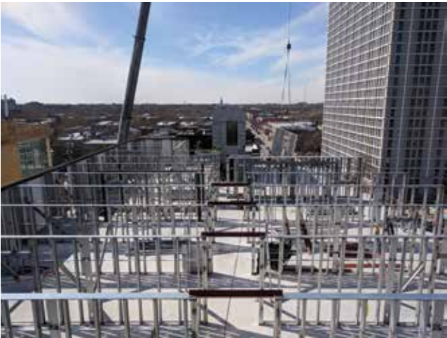
Pre-fabricated, structural CFMF wall panels. Courtesy of Bear Construction Co.
