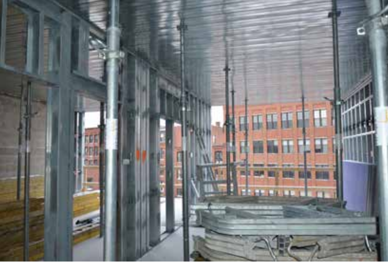
Shored long-span steel deck construction.
