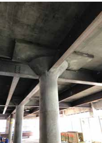
Figure 5. The underside of roof slab reinforced with additional non-composite steel beams.
