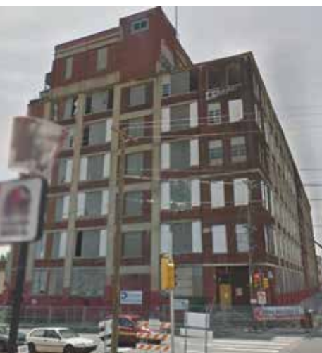
Figure 2. Apex Hosiery Company Building located in Philadelphia – prior to renovation.
