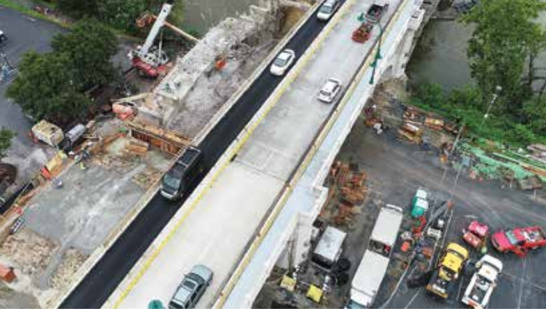
Staged construction showing the superstructure removed (left side of bridge), temporary paved lane (center) and new construction (right side of bridge).
