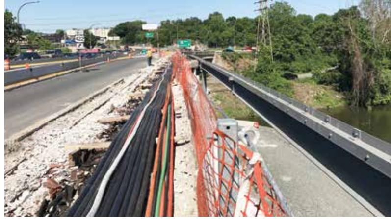
The design incorporated a way to excavate fiber optic lines from the existing sidewalk, temporarily support the lines on the side of the bridge via a temporary support, reconstruct the bridge deck, and cast the utilities back in the new sidewalk including a vault to access splices.
