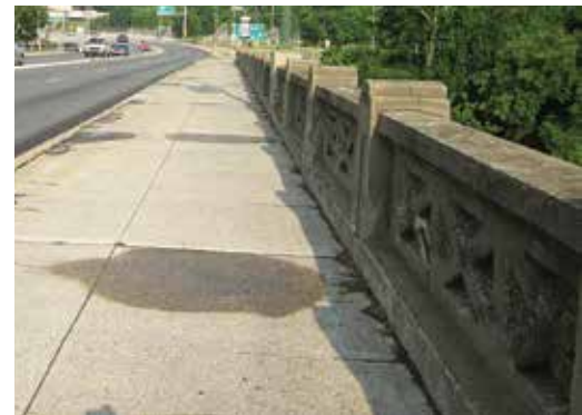
The most notable change is the reconstruction of the reticulated balustrades (right) with outlooks, which were closed in the 1950s due to deterioration.
