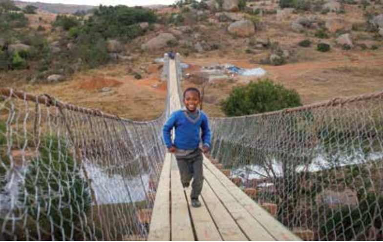
The completed Edlangeni Footbridge provides safe access for children to attend school year-round. Courtesy of Madison Sankovitz.
