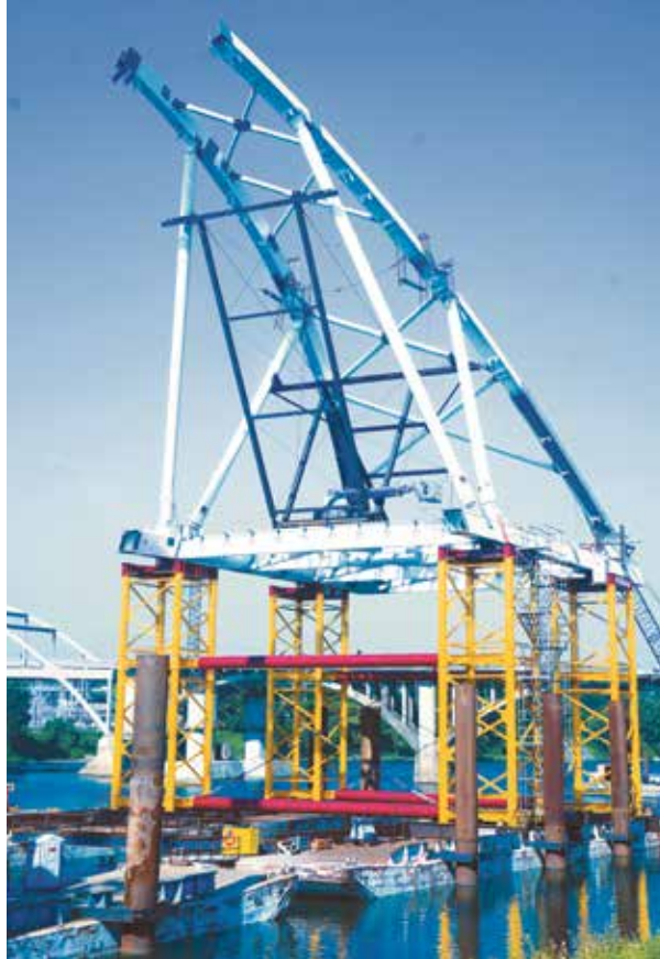
Arch span during erection with adjustable temporary struts.
