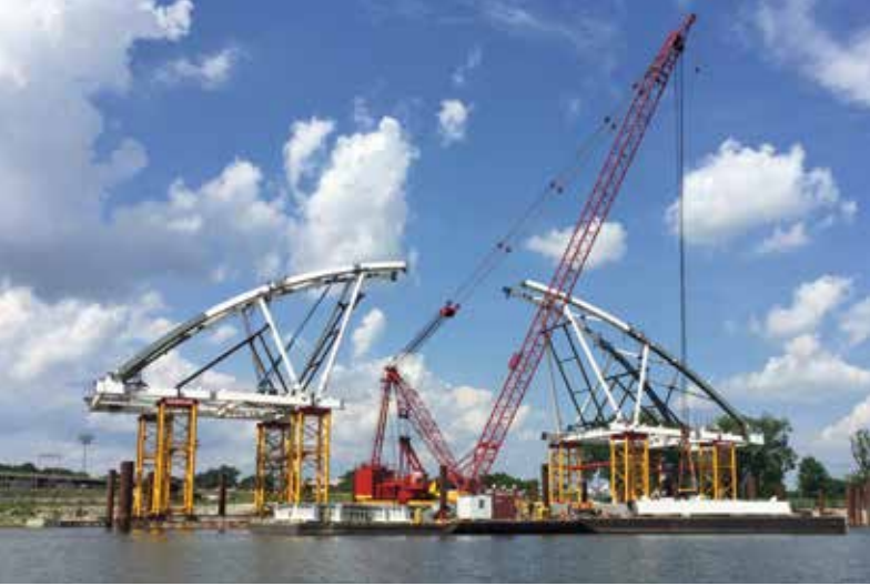
Arch span prior to closure.
