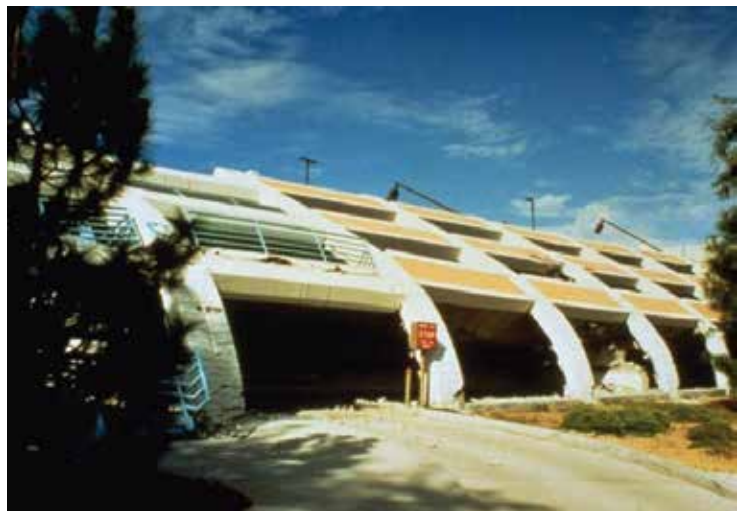
Figure 1. Precast concrete garage failure at Cal State Northridge. Courtesy EERI.
