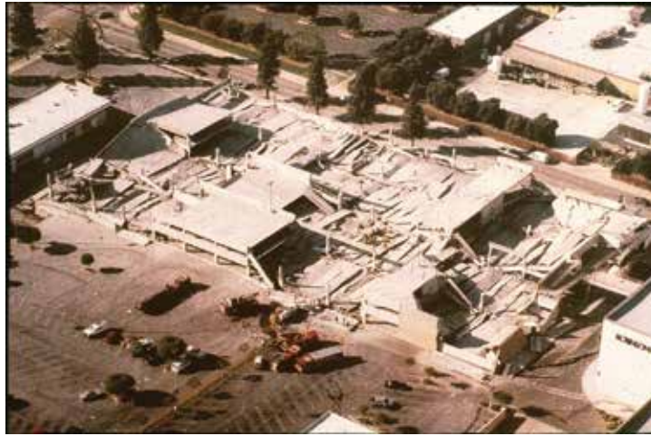
Figure 2. Failure of precast garage at the Northridge Fashion Center. Courtesy EERI.
