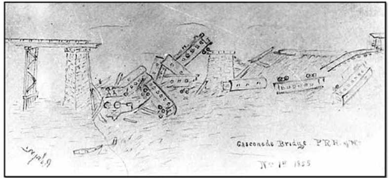
Sketch of disaster, note temporary bent for approach and masonry piers.
