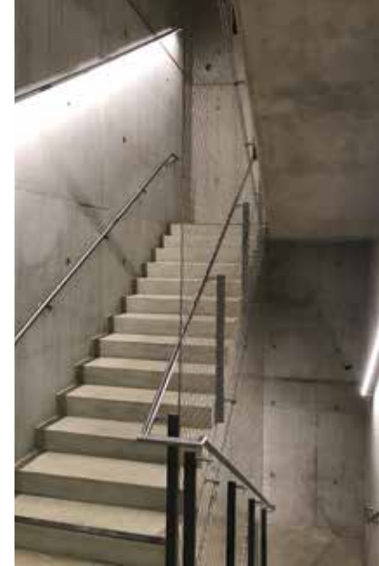
View of completed stair with coordinated wall formwork. Courtesy of Payette.
