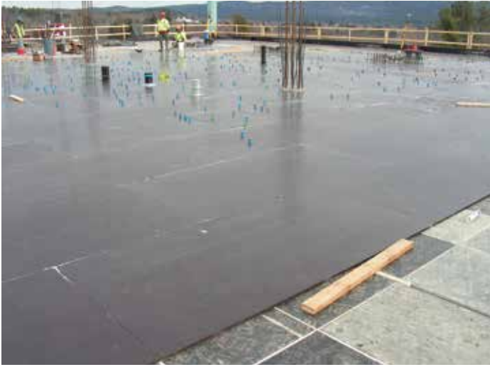
Formwork and HDO panels being placed for architectural concrete.
