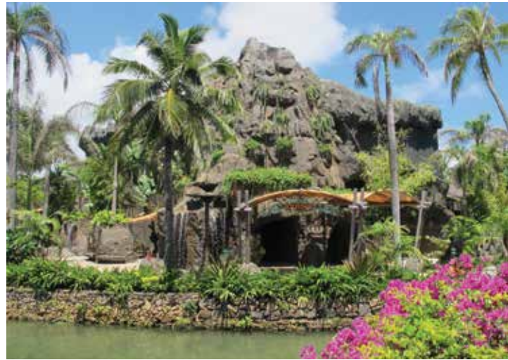
J.M. Williams & Associates, Inc. was an Award Winner for its Polynesian Cultural Center Renovation project in the 2018 Annual Excellence in Structural Engineering Awards Program in the Category – Forensic/Renovation/Retrofit/Rehabilitation Structures over $20M.
