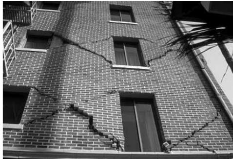
Figure 1. Cracking in masonry wall after an earthquake.
