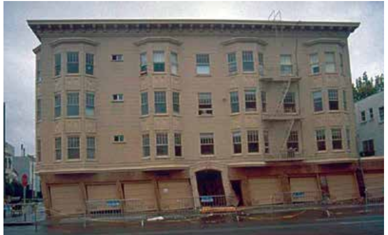
Figure 1. Building damaged in 1989 Loma Prieta earthquake. Courtesy of Raymond B. Seed.
