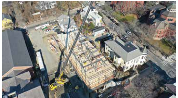
Drone photo of the structure under construction.
