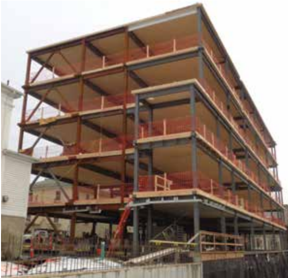
Structure at north elevation.
