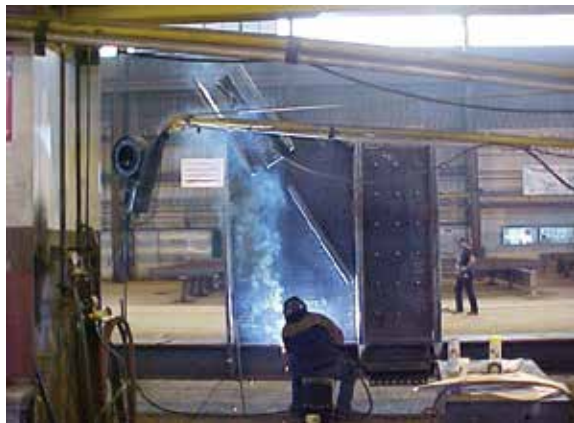
Figure 2a. Large gusset plate being fabricated.
