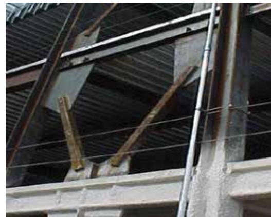
Figure 2b. Very large gusset plate installation.
