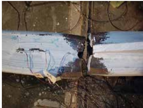
Figure 1 a. Net section fracture occurring at ductilities less than expected.
