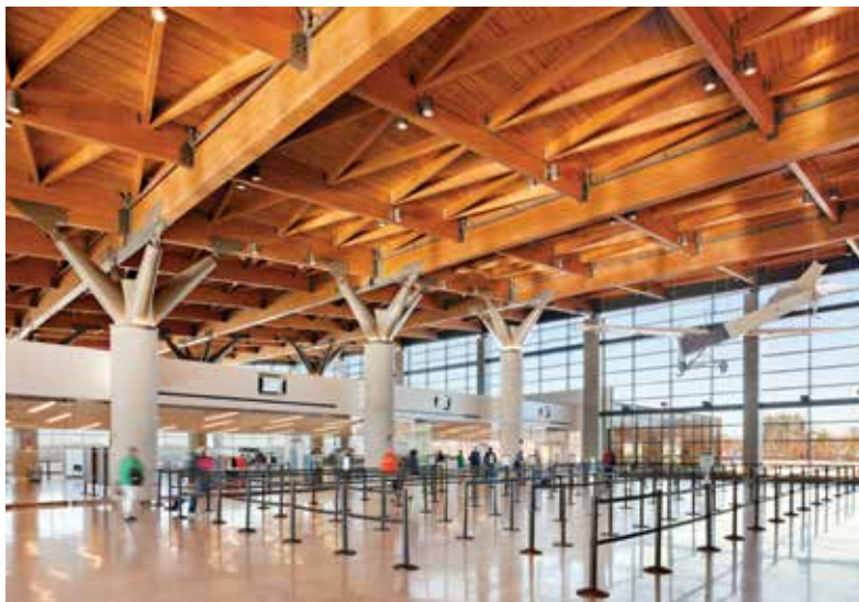
Portland Jetport's glulam timber roof structure. Courtesy of Robert Benson Photography.
