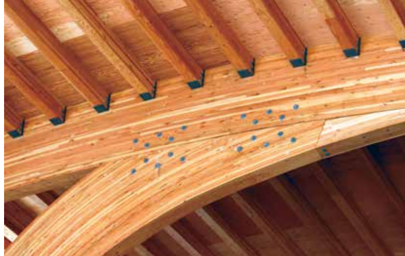
Mystic Seaport Exhibition Building's glulam timber connections transfer structural loads in bearing with minimal exposed bolts and steel hardware.
