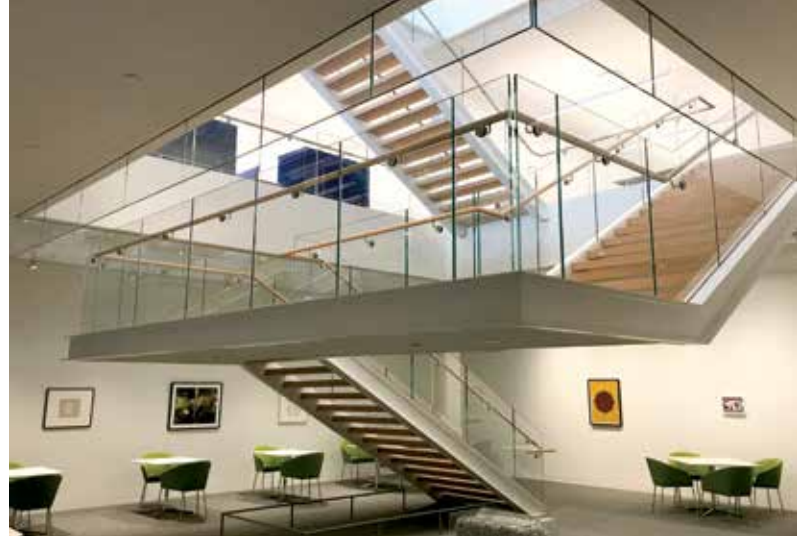
Figure 3. Free-floating interior stair between 3 rd and 4 th floor.
