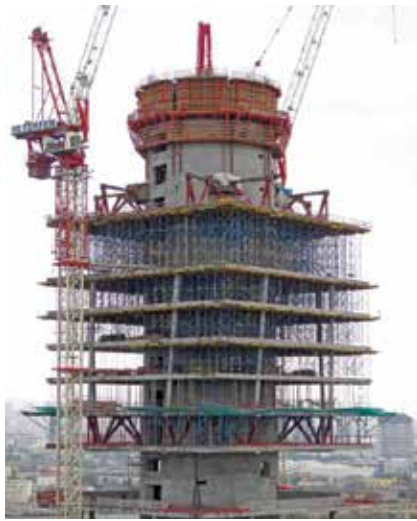
Figure 4. Shoring the transfer system. Courtesy of Tekfen Construction.
