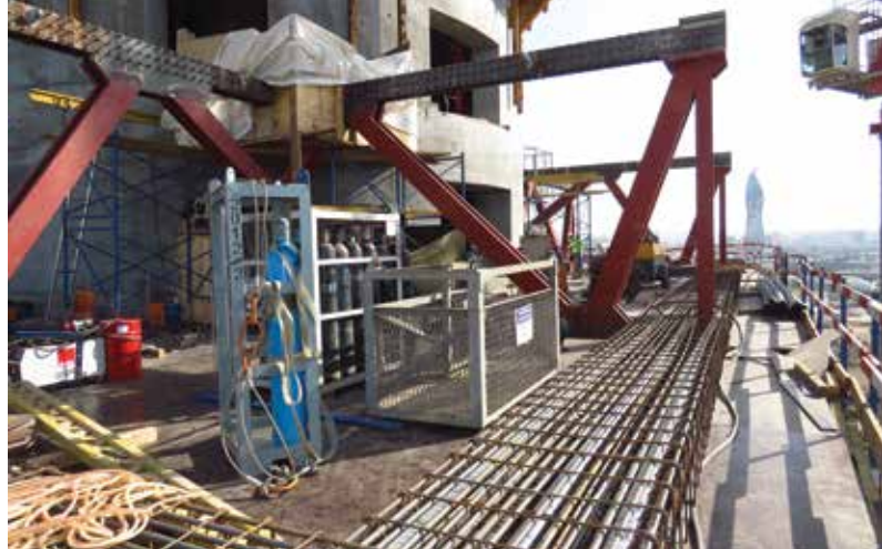
Figure 3. Transfer truss construction. Courtesy of Tekfen Construction.
